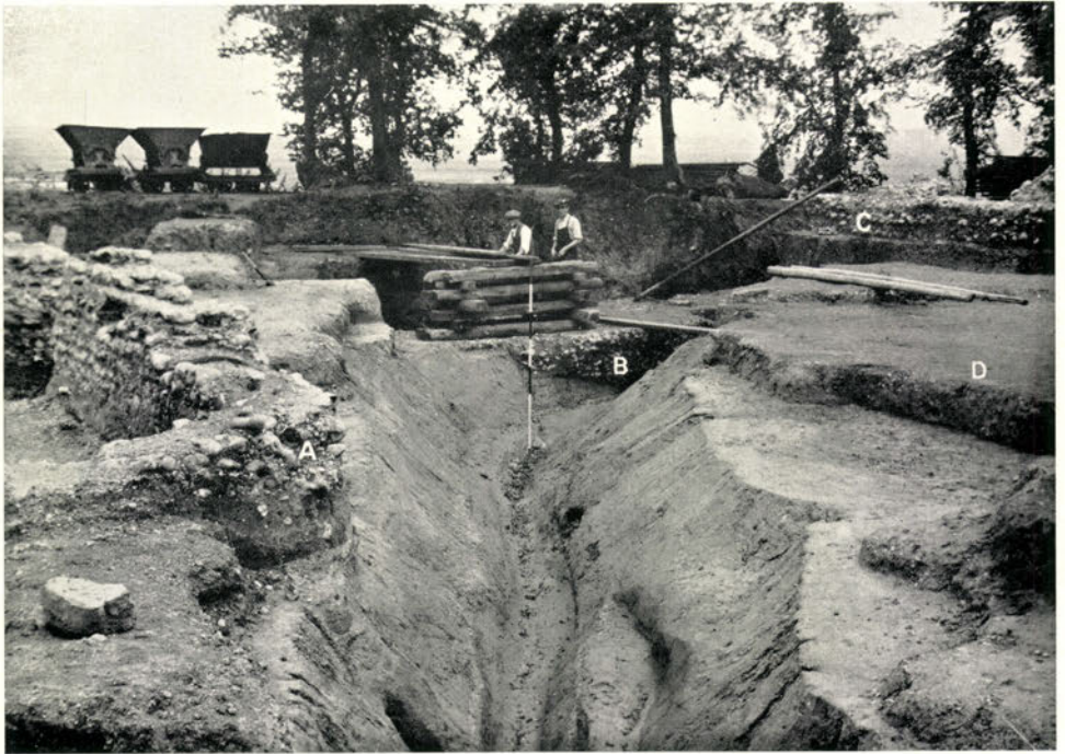
Fig. 2. A. S.W. angle of 2nd house, Site III; B. foundation of E. wall of fort, passing over inner ditch, pp. 19, 23; C. N.E. angle of chapel, p. 34; D. mixing floor, p. 10
