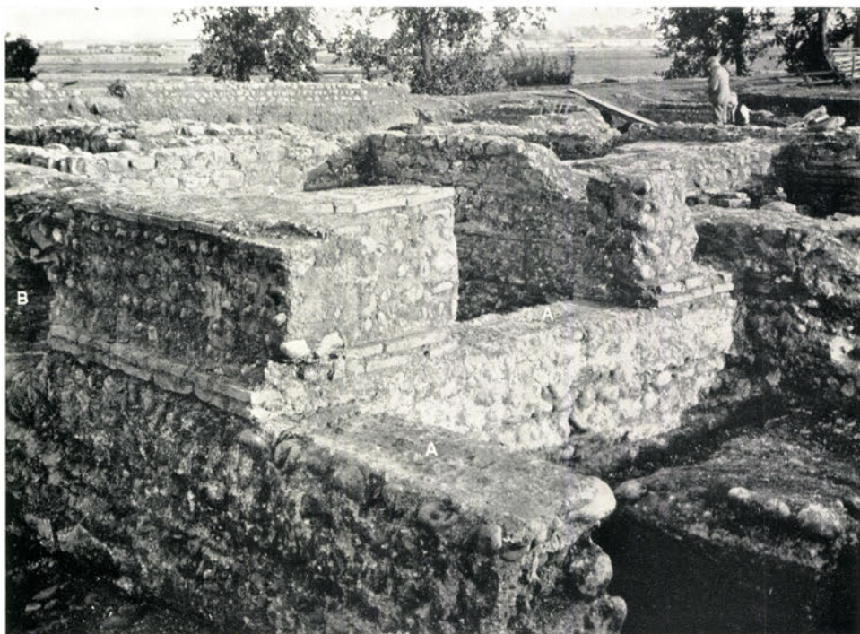
Fig. 2. Site III. A, A, doorways into room 7, 2nd house, p. 17; B, inserted opening in N. wall of room 8, 2nd house, p. 17
