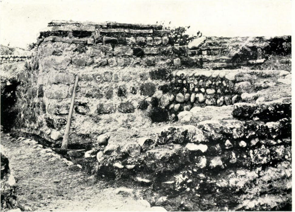
Fig. 1. Site III. A. S. wall of room 15, 1st house, p. 13; B. W. wall of room 16, 2nd house, p. 15; C. wall of room 1, bath building, p. 24
