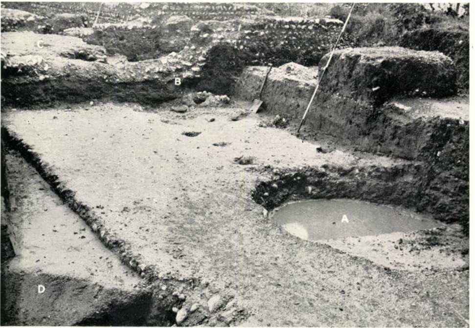
Fig. 2. Foundation of E. wall of fort looking N., p. 23. A. pit 26, p. 33; B. S. wall of 2nd house, Site III; C. surface of foundation of E. wall of fort at higher level, p. 23; D. N. side of inner ditch, p. 20
